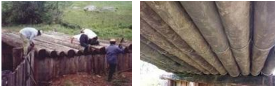
Fig. 5. Launch of timber beams
