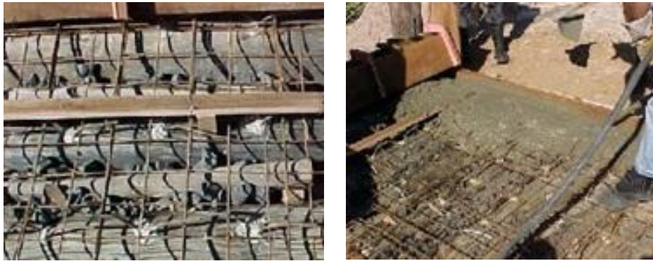
Fig. 9. Details of final armor and beginning of concreting
