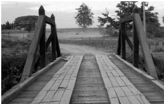
Fig. 1. Typical deck sawn timber [5]
