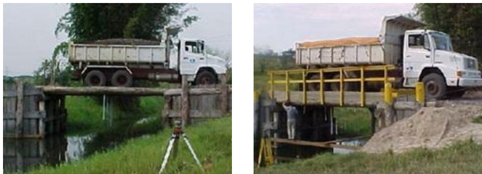
Fig. 10. Load test on the timber beams and the completed bridge
