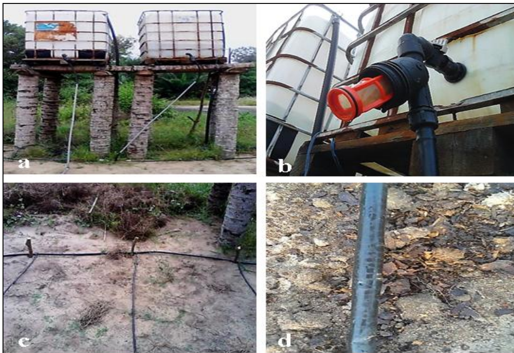
Fig. 4. Drip irrigation system consisting of (a) tanks of 1000 l, mounted on supports made of coconut stems 2 m high, (b) filter, (c) ramps and (d) drippers on a ramp
