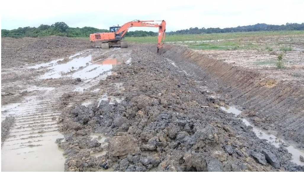
Fig. 4. Construction of erosion control channels
