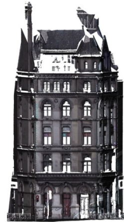
b) Feature based registration (6.7mm error) – 44 Westmoreland St. with Trimble data
